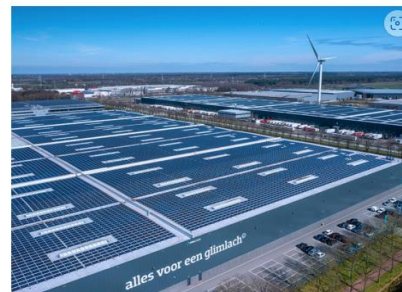
Prologis Tilburg Aerial photo with windmill in the background
